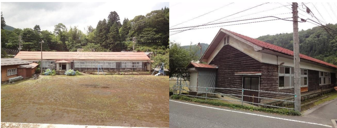
Figure 5: The targeted abolished school (left) and the school made of wood (right).
