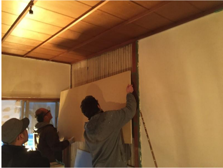
Figure 4: Renovation in the PBL challenge.
