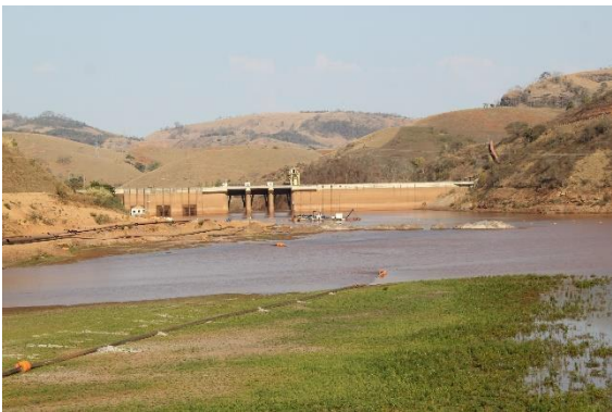
Figure 8 - Risoleta Neves Hydroelectrical power plant. It is possible to see its floodgates open since the day of the burst. Picture took showing the area of the dam that is empty.
