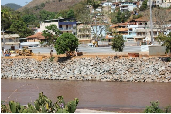
Figure 6 - Main square under reconstruction in Barra Longa.
